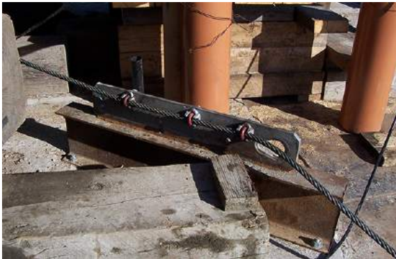
Deadman anchor used to hold 3/4 inch safety cable
