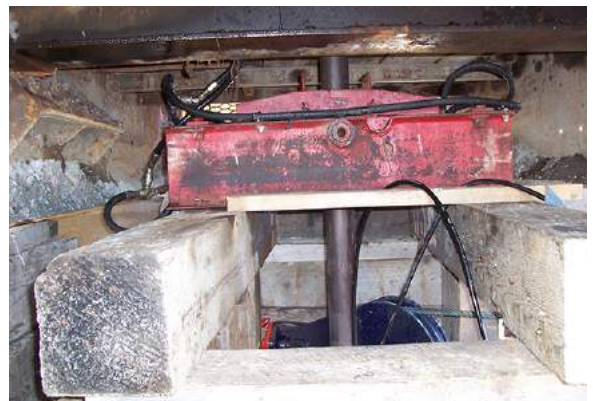
Foot clamp holding HQ drill rods
