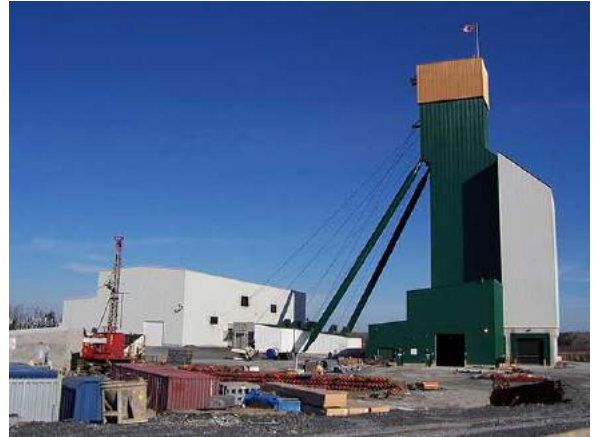
Project site with pilot hole situated beneath diamond drill (shown on left)
