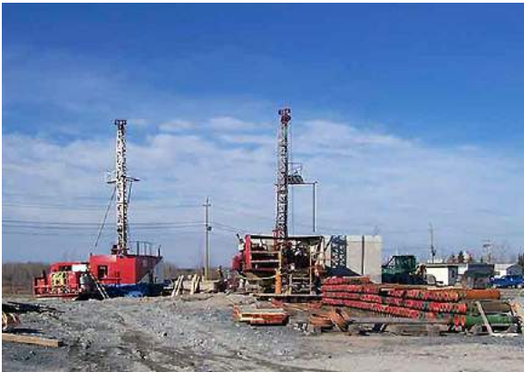
Drilling NQ grout holes in proximity to pilot hole
