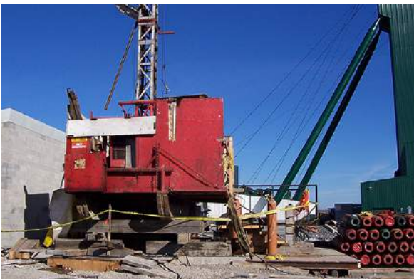
Diamond drill elevated above pilot hole collar
