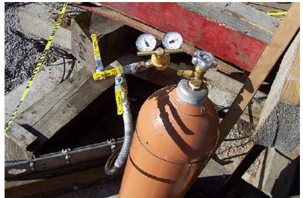
Nitrogen tank with regulator for inflating packers
