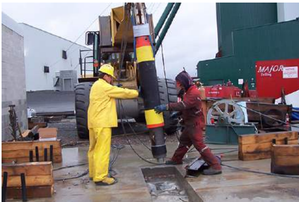
280 mm diameter inflatable packer assembly installation at collar of pilot hole
