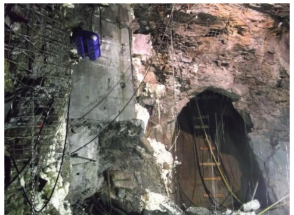
Dry tunnel excavation
