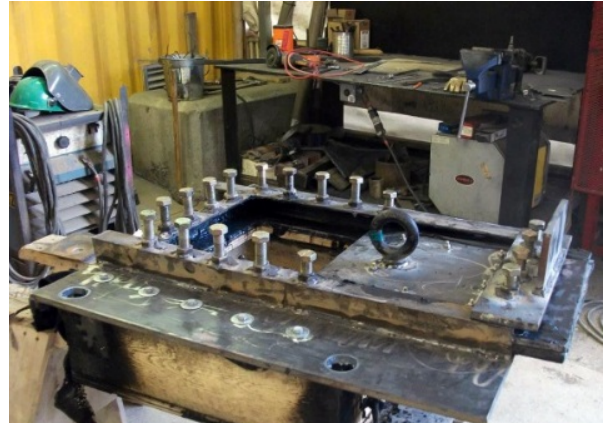
Water control gate fabrication
