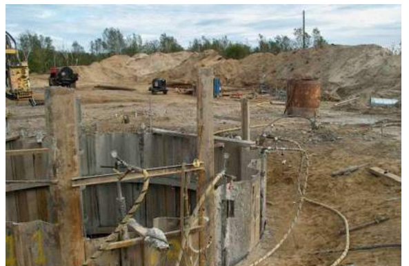
Cement grouting through external grout pipes
