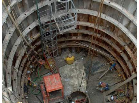
Sealing quicksand inflows at sheet pile – rock interface
