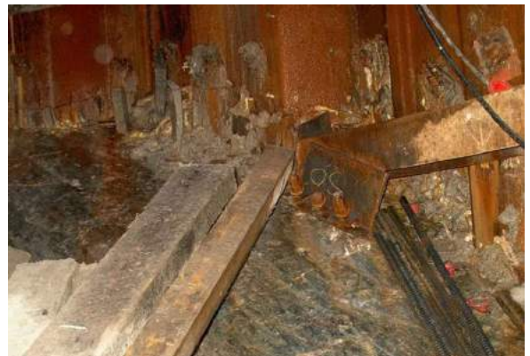
Sealed sheet piles at bedrock contact
