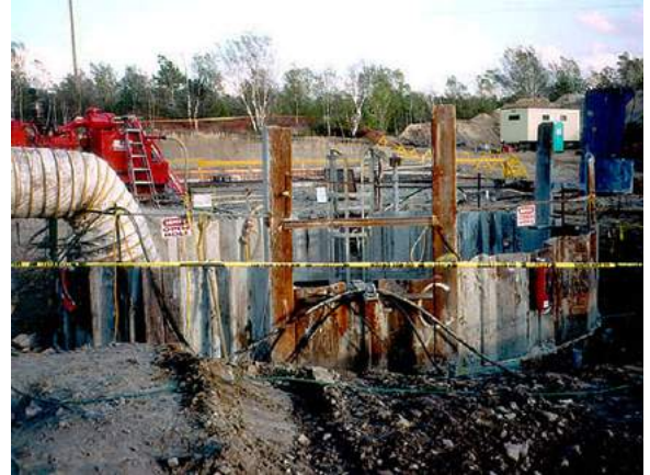
Shaft Collar with sheet piles
