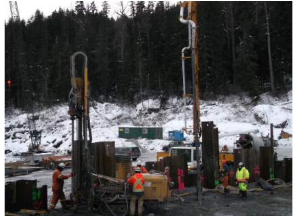
Drilling and grouting at Stage 2 cofferdam
