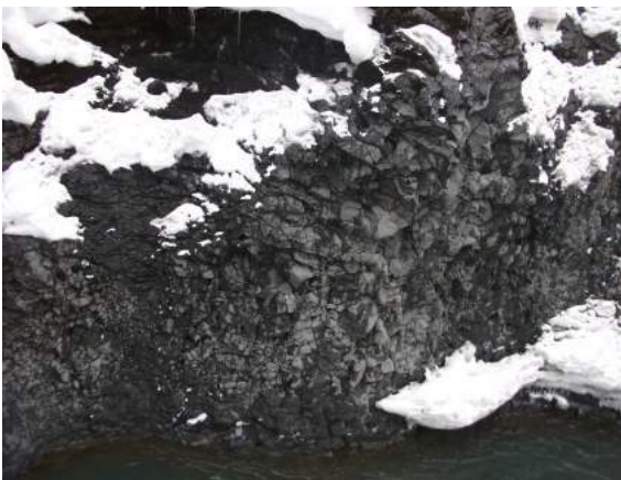
Porous rock formation beneath cofferdam
