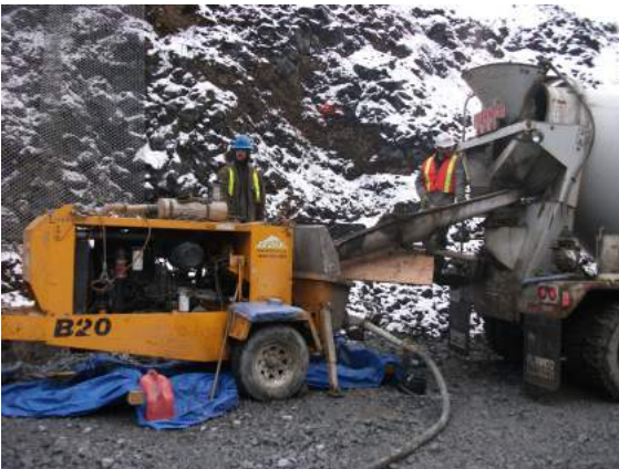
Mayco B20 concrete pump in operation
