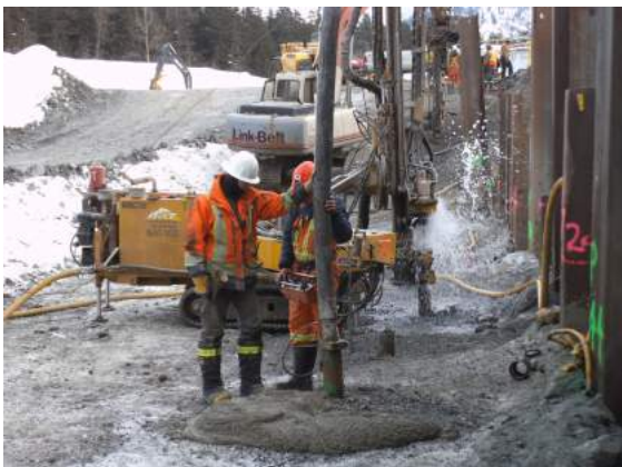
Drilling and grouting at Stage 2 cofferdam
