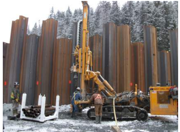
Drilling grout holes adjacent to cofferdam
