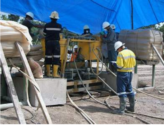
Typical grout plant setup at surface
