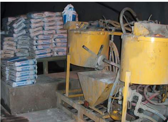
Typical grout plant setup underground
