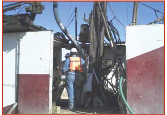
Excellon Resources, Platosa Mine, Mexico Deep hole drilling and high-volume cement grouting operations were used to seal water-bearing rock formations and successfully recover a flooded underground silver mine.
