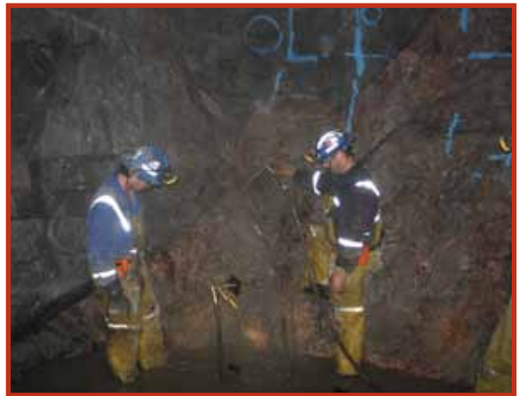
Rio Tinto, Diavik Diamond Mine, Canada Cement grouting methods are used to fill water-bearing fractures and reduce the potential for high-volume groundwater inflows prior to underground mine development operations.
