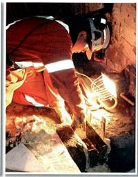
Grouting work consisted of several stages that included shallow chemical grouting to a depth of 0.6 m, deeper chemical grouting to a depth of 1.2 m, followed by cement grouting with holes drilled to a depth of 4 m. The initial chemical grouting work resulted in an immediate and significant reduction in water inflow entering the shaft although water was subsequently encountered
