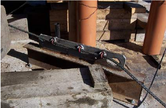
Deadman anchor used to hold 3/4 inch safety cable
