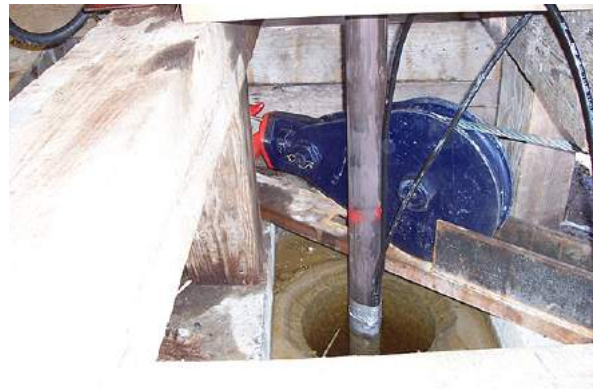
Sheave wheel for 3/4 inch safety cable at collar of drill hole with packer inflation hoses attached to HQ drill rods
