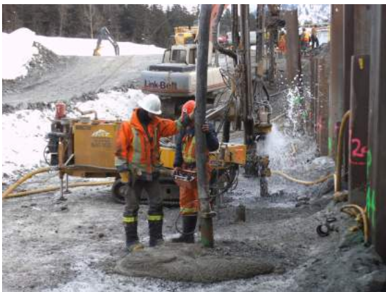
Drilling and grouting at Stage 2 cofferdam
