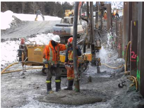
Drilling and grouting at Stage 2 cofferdam
