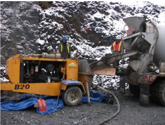
Mayco B20 concrete pump in operation
