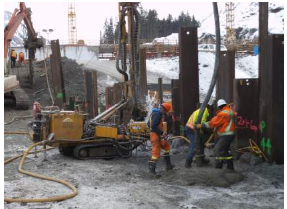
Drilling and grouting at Stage 2 cofferdam
