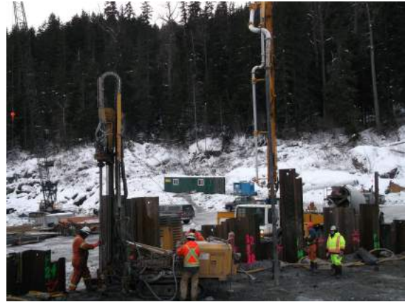
Drilling and grouting at Stage 2 cofferdam
