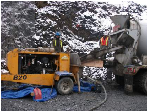
Mayco B20 concrete pump in operation
