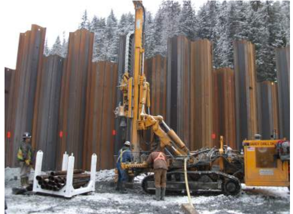
Drilling grout holes adjacent to cofferdam
