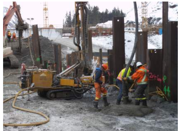
Drilling and grouting at Stage 2 cofferdam
