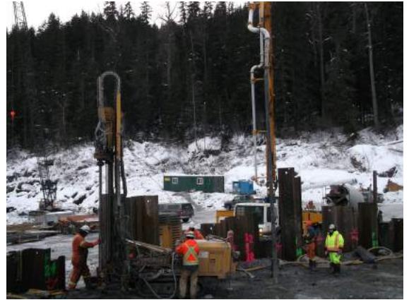
Drilling and grouting at Stage 2 cofferdam
