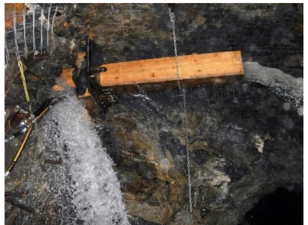
Water control gate and water diversion sluice
