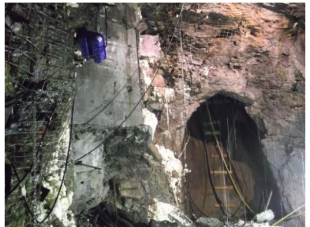
Dry tunnel excavation
