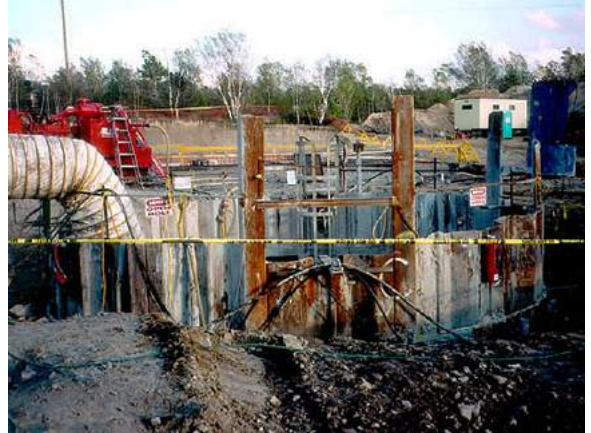
Shaft Collar with sheet piles
