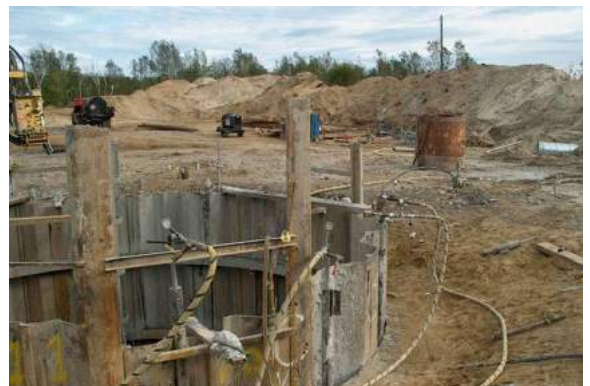
Cement grouting through external grout pipes
