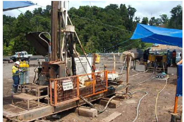
Diamond drill in foreground, grout plant in background
