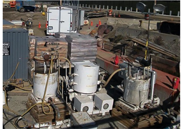
Grout plant setup adjacent to shaft grouting location
