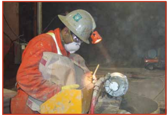
Sifto Salt, Goderich Mine, Ontario Chemical grout, applied as spray foam, was used to seal a five meter high by eight meter wide underground ventilation bulkhead. A layer of cement grout (in the form of spray foam) was applied over top for fire protection purposes.
